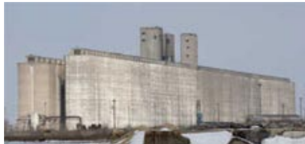
On the market: A 1950s grain elevator in Wichita that can't be used as a grain terminal.
